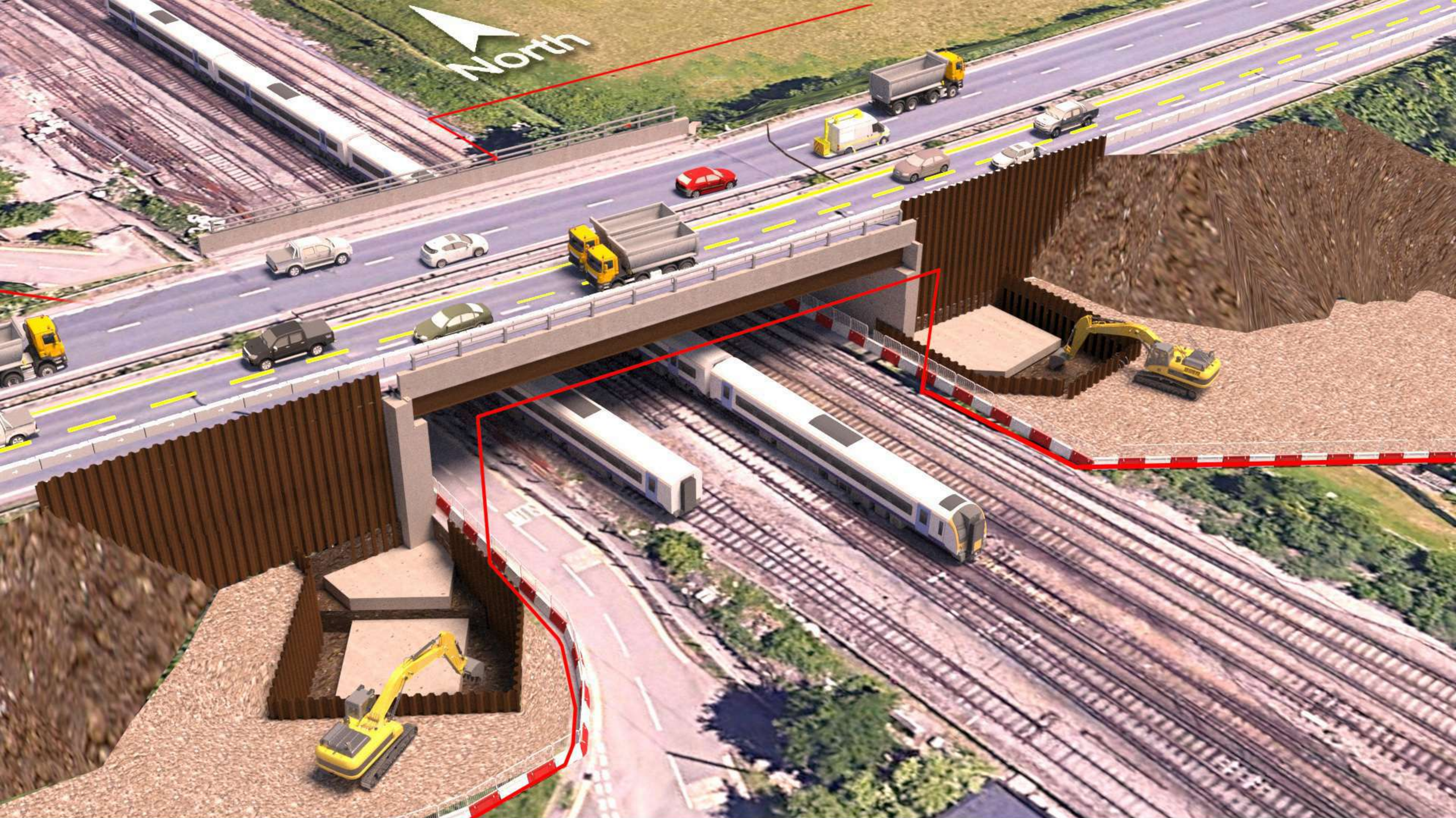
Airport Way Rail Bridge
