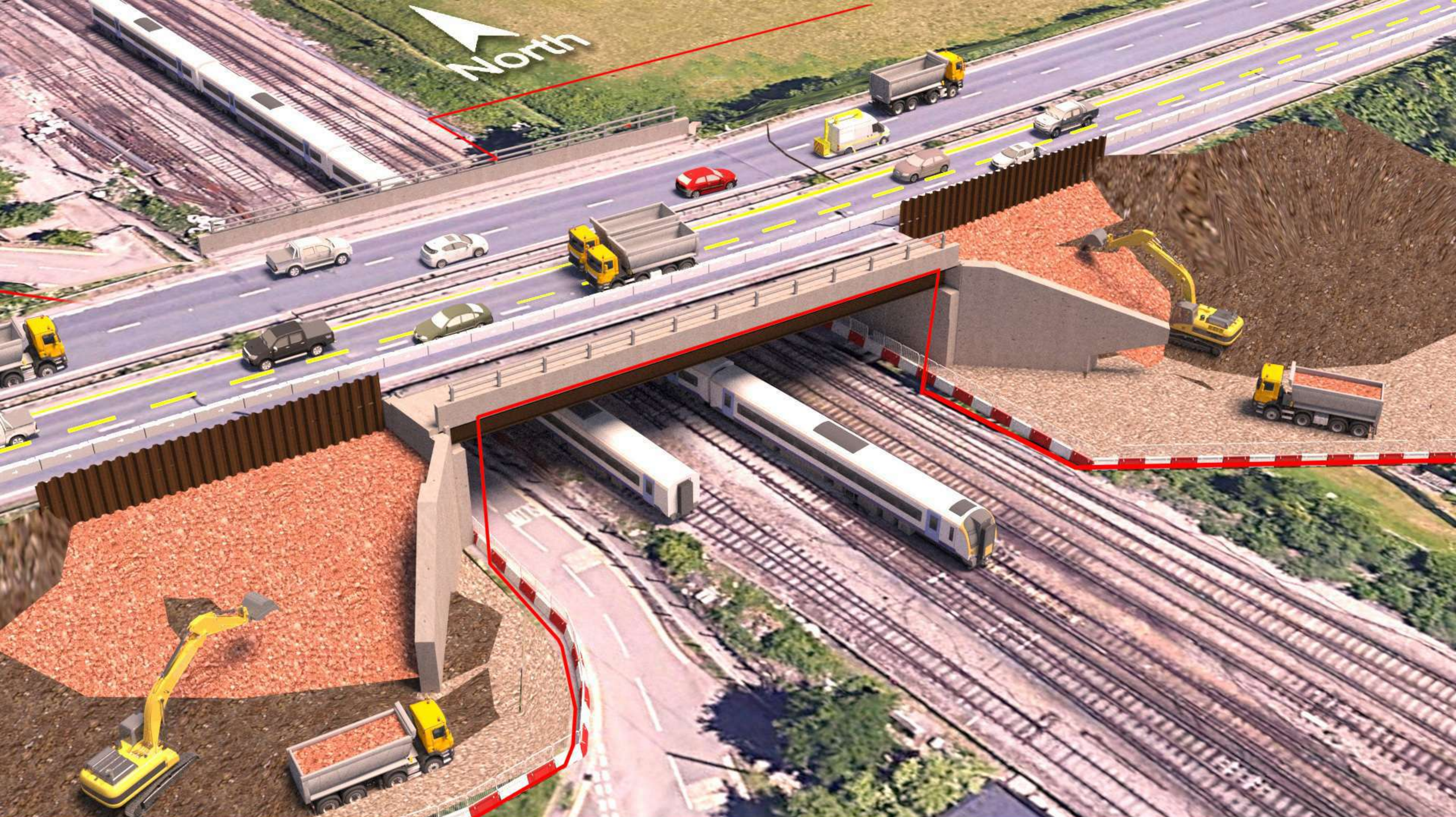
Airport Way Rail Bridge
